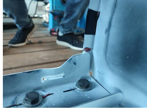
试验后状态 State after test
